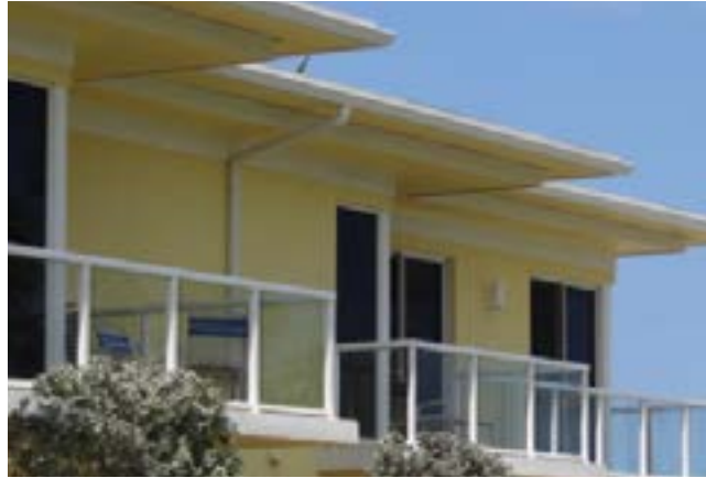
(22) Cantilevered roof with overhang
