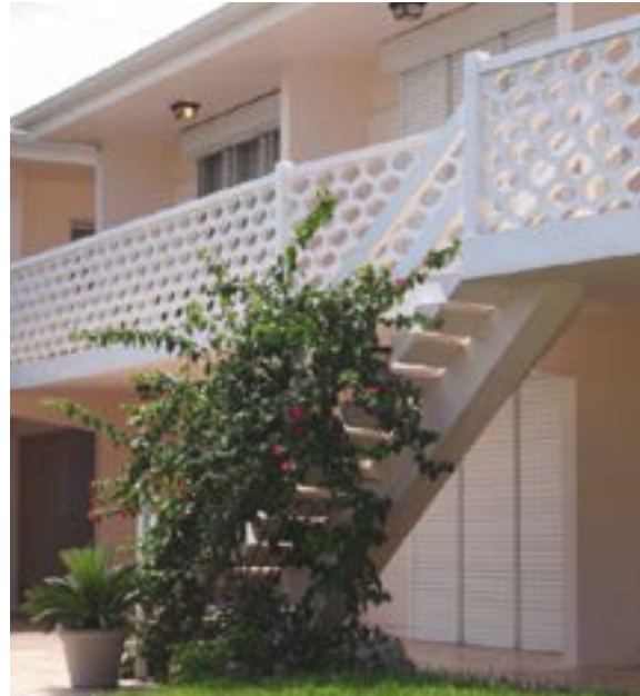
(18) Outdoor corridor with floating Staircase
