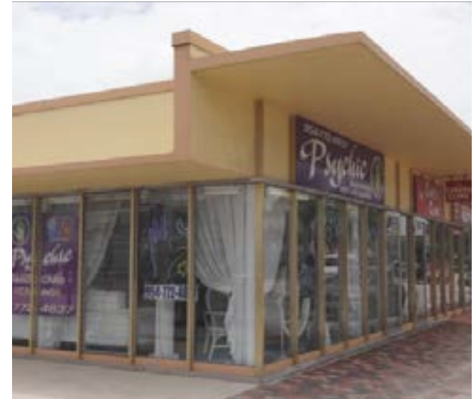
(19) Parapet roof with eyebrow
