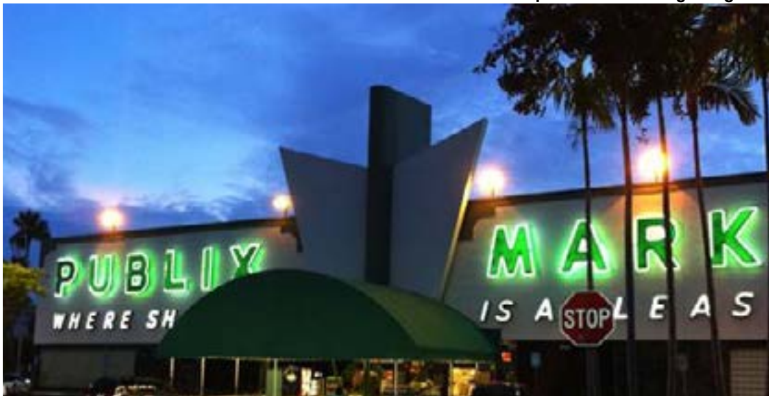
Horizontally supported neon letters below and reverse channel illuminated letters above on wall as part of the building design
