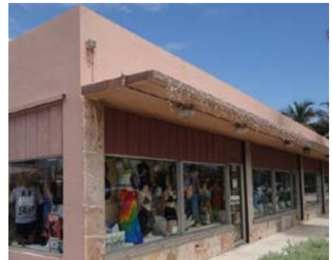
(19) Parapet roof with eyebrow
