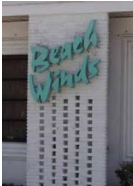
4. Inverted channel letters on architectural masonry sign board.
