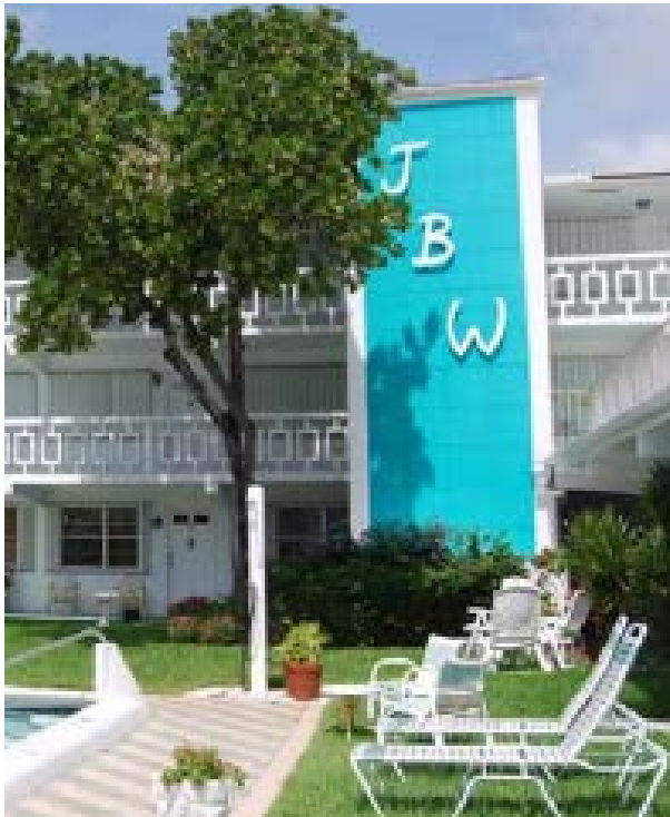
Reverse channel letters horizontally attached to architectural masonry wall scored to look like tiles
