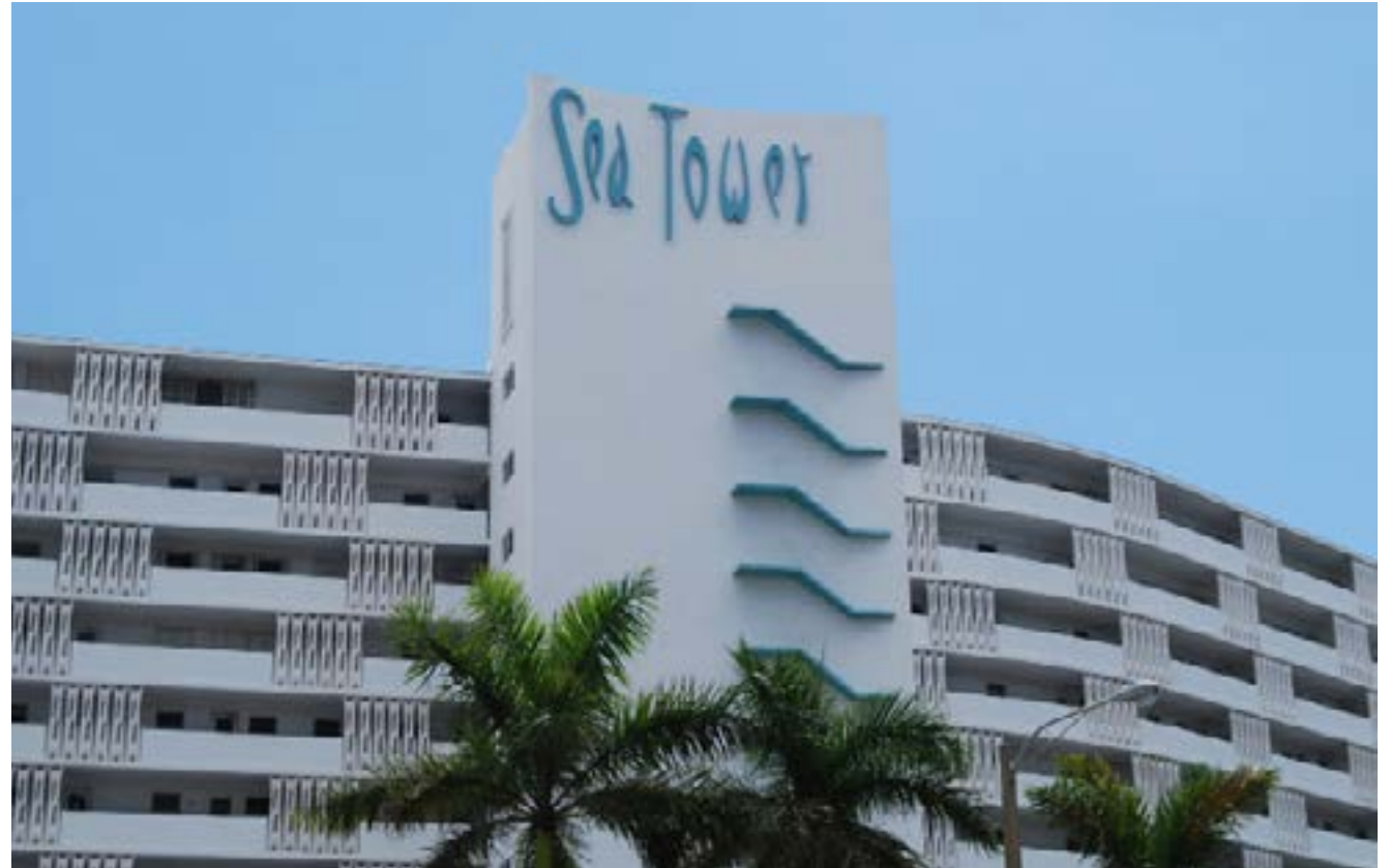
Horizontally supported on wall as part of the building design
