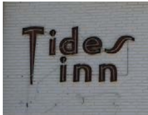
b. Exposed neon lighting on architectural masonry support
