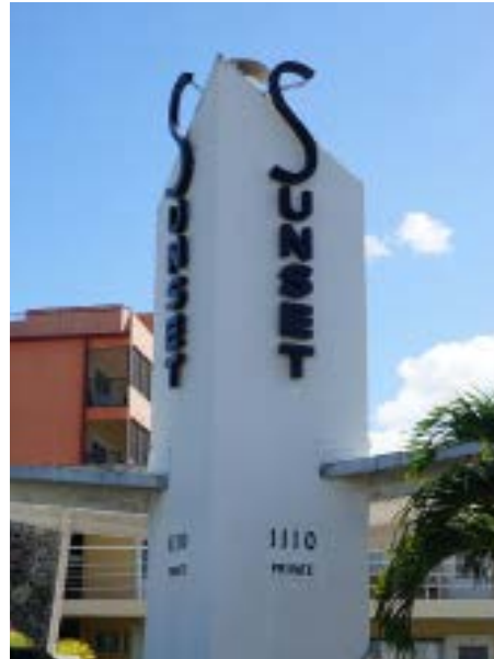
3. Masonry monument support.
