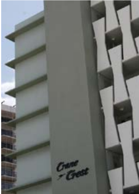
2. Sign on architectural masonry support with horizontal projecting letters.
