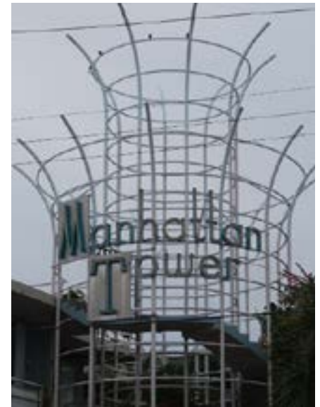
1. Multiple steel tube structural support
