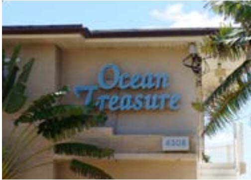
Horizontally supported individual reverse channel lettering
