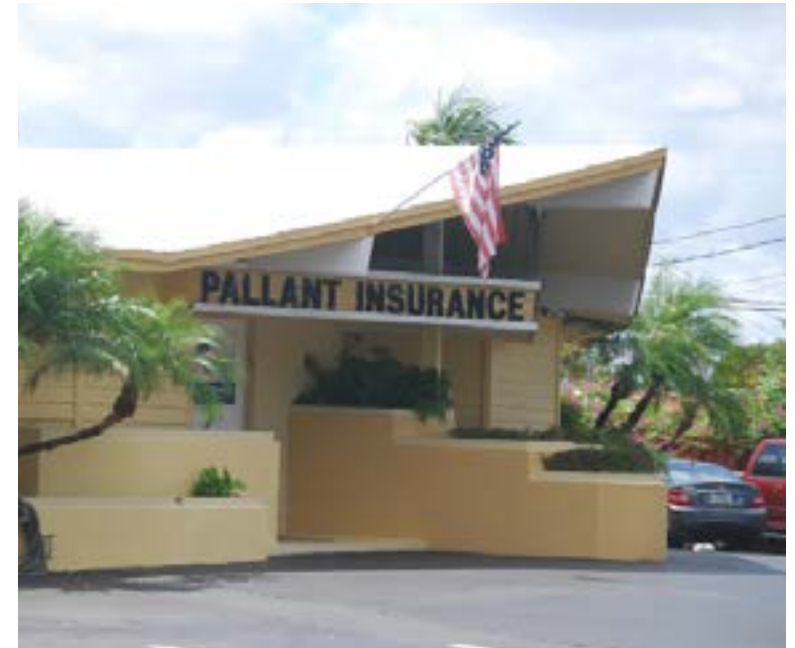
4. Individual reverse channel lettering on signboard integrated with building.
