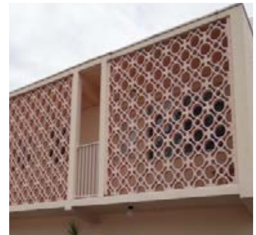
(23) Shading devices, catwalk, with Brise Soleil
