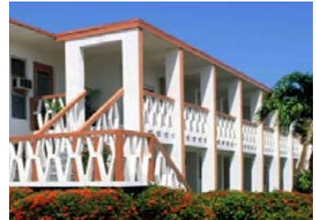
(3) Roofs and outlining trim
