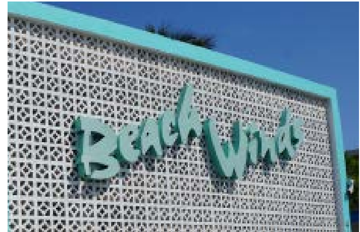
Reverse channel letters horizontally attached to architectural masonry wall
