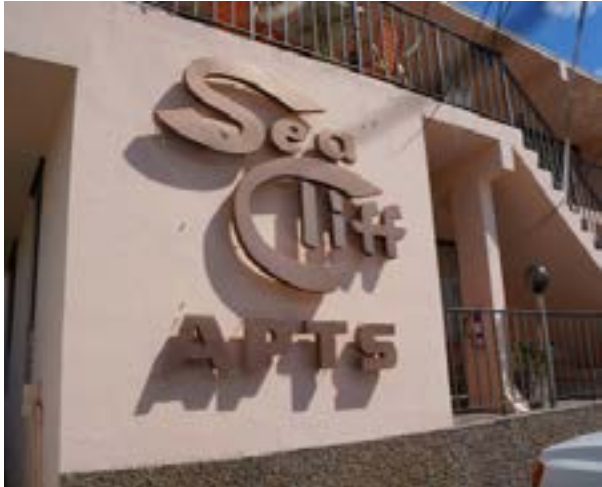
Reverse channel letters horizontally attached to architectural masonry wall
